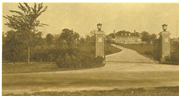
(Braebourne Estate as seen from Riverside Drive, constructed in 1922)
